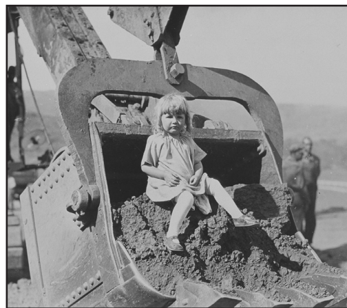
Beverly Boulevard grading, 1924. Photo: PPHS Collection/Zola Clearwater Archive
