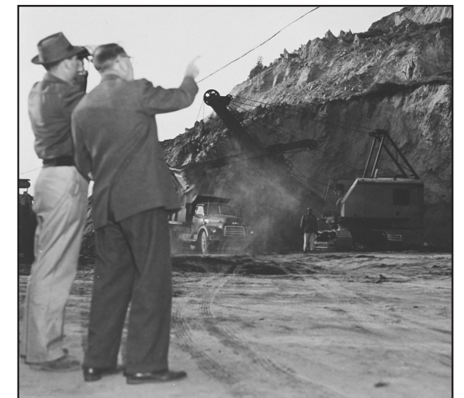
Killer landslide closing PCH, 1958. Photo: PPHS Collection/Zola Clearwater Archive
